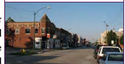
The above illustration and photo illustrates the preferred variation in roof lines.
