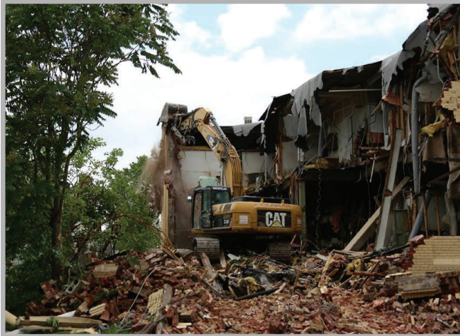
June 2, 2015 demolition progress Main Street Apartment Building -- W. Main Street
