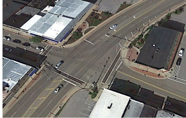
Channelization at Intersection
