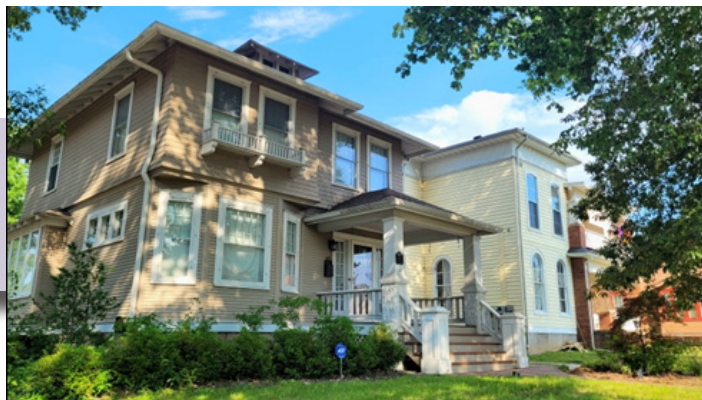
Falline House, 120 North Aurora
