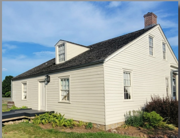
The D.D. Collins House has traditional wood clapboard siding that has been painted in a period appropriate color.
