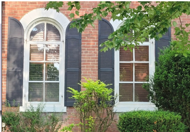
Note the original wood windows featuring appropriately sized and mounted shutters. The shutters, if closed, would completely cover the window opening and match the window's size and shape.
