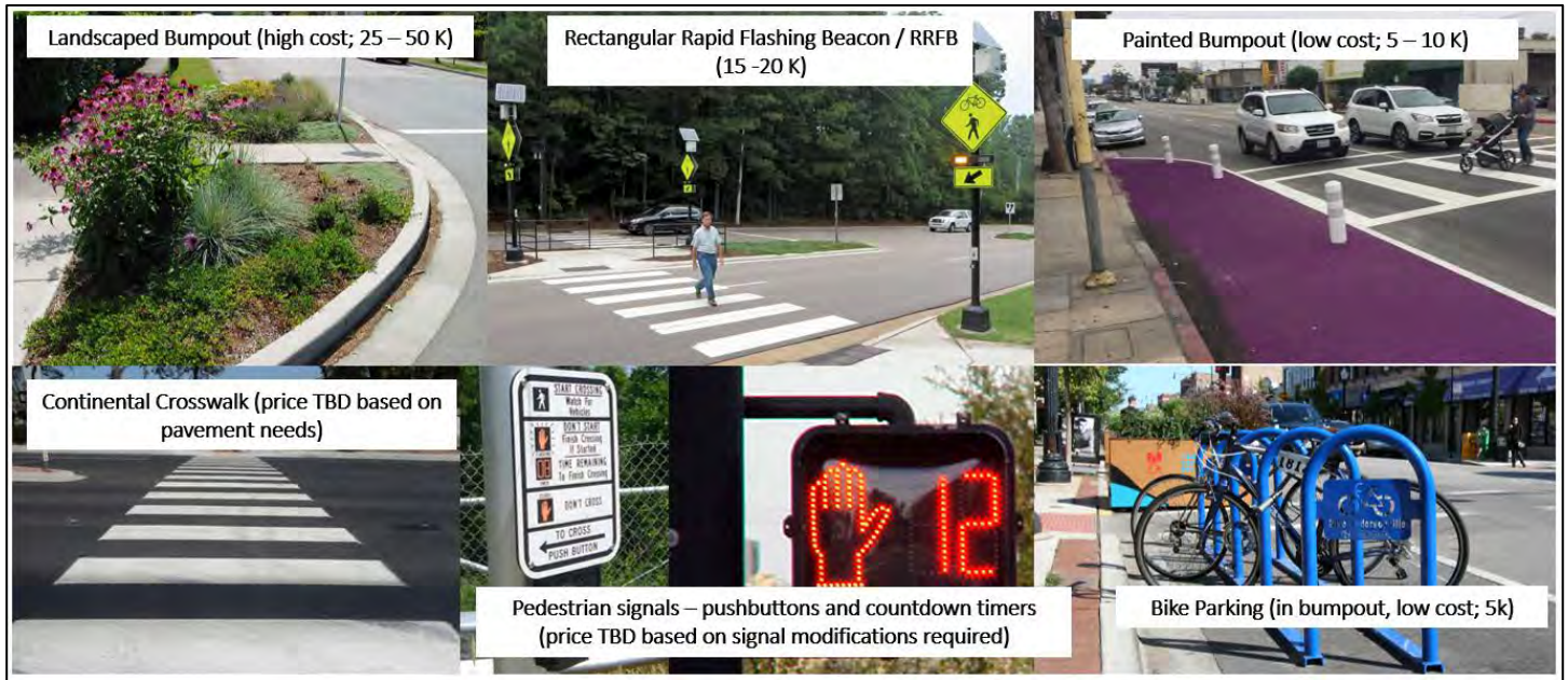
Proposed Slow Zone Crossing Treatments – examples from multiple locations (cost is only to install, should develop maintenance plan based on lifecycle of materials selected for implementation)
