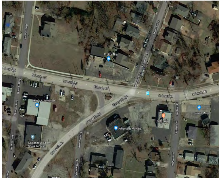
Existing intersection at St. Louis Road and Caseyville Road
