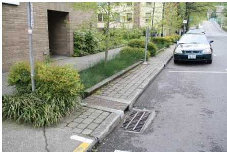
Example of a BMP where stormwater can infiltrate in a planted area. Especially in areas with on-street parking, BMP's should provide space for passengers to disembark.
