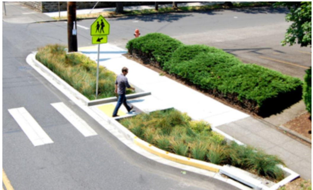
Example of a bulb out with landscaping. The bulb out also provides space for street tree plantings.
